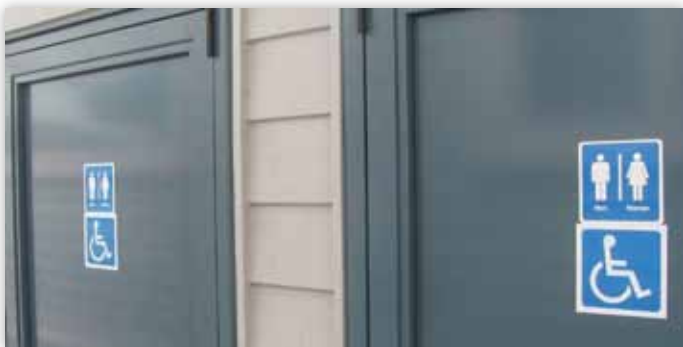
2 wheelchair loos in the new building
