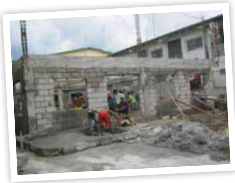
The progress on the first floor of the House of Love and Compassion. There will be a second floor for classrooms of SPED High School Deaf
